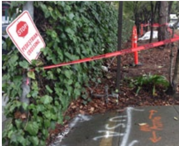
CPMC has started installing light bollards along 14th Street
