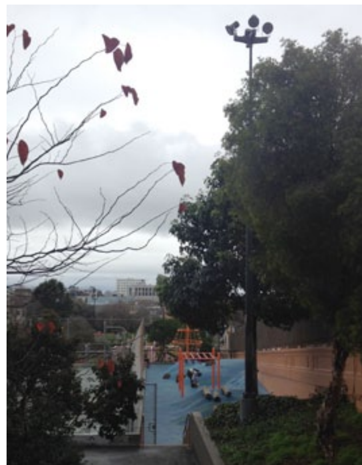
A tree is blocking some of the light that should be illuminating the youth play area
