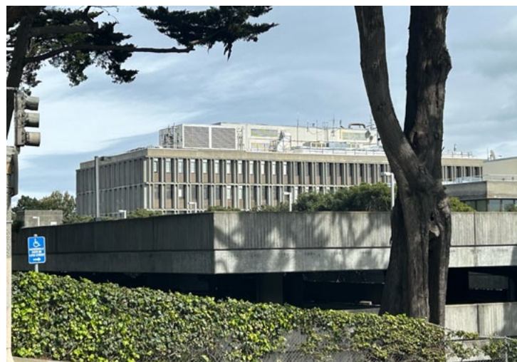
From Castro and 14th CPMC's noisy HVAC units are visible on the roof.
